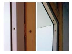
9 It is important to shim properly as you would with a door or window. Run additional fasteners (not provided) through exposed composite and into frame lumber.
