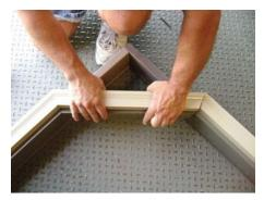
5 Press down firmly with palms or use rubber mallet to lock nosing onto aluminum cap.
