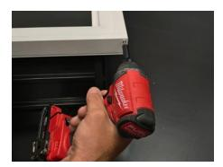
6 Install 1" stainless steel corner screw into predrilled holes using a #1 square drive bit.
