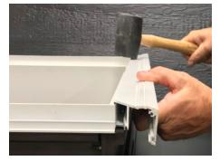
5 Press down firmly with palms or use rubber mallet to lock nosing onto aluminum cap.
