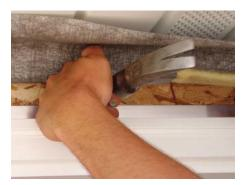
8 Fold back aluminum nailing fin. Fasten through pre-punched holes.
