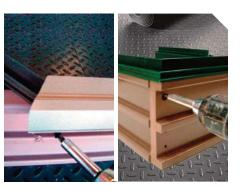
3 Locate pre-drilled holes and install 8 each 1-5/8" black, course thread screws.
