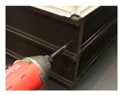
B Locate pre-drilled holes and install 8 each 1-5/8" black, course thread screws.
